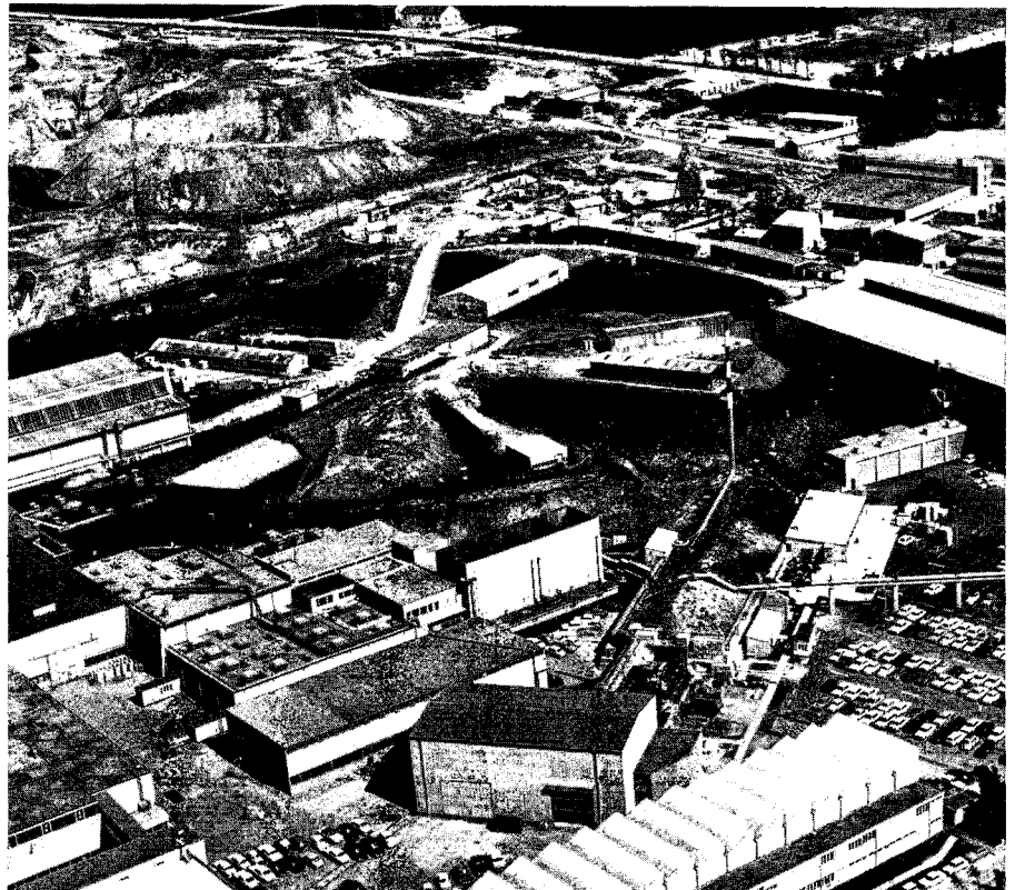
An aerial view of part of the CERN site. The wheel shape of the proton synchrotron itself is fairly obvious and, pointing from it towards the bottom of the picture, is the tunnel housing the neutrino beam-line. The large new building (bottom centre of the picture) is the one which will house Gargamelle.
